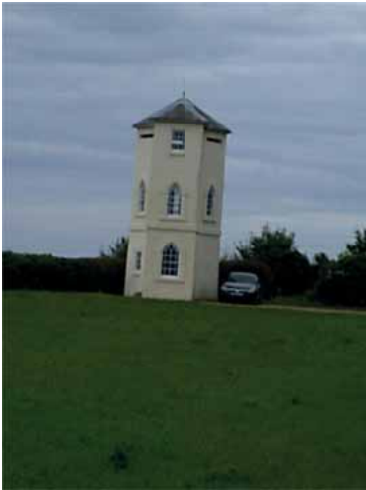
The Leaning tower of Mont Ube
