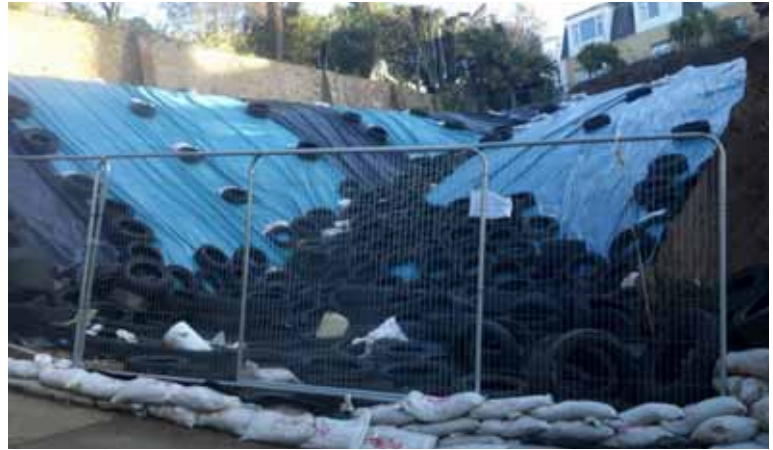
Landslide on College Hill
