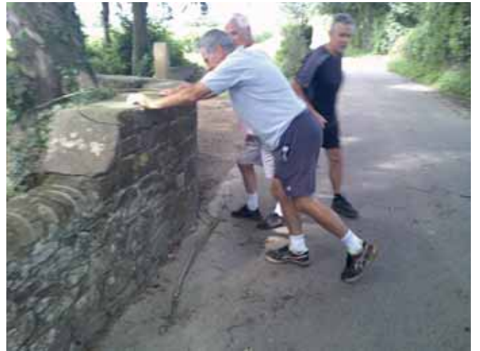
I must stop this wall from falling
